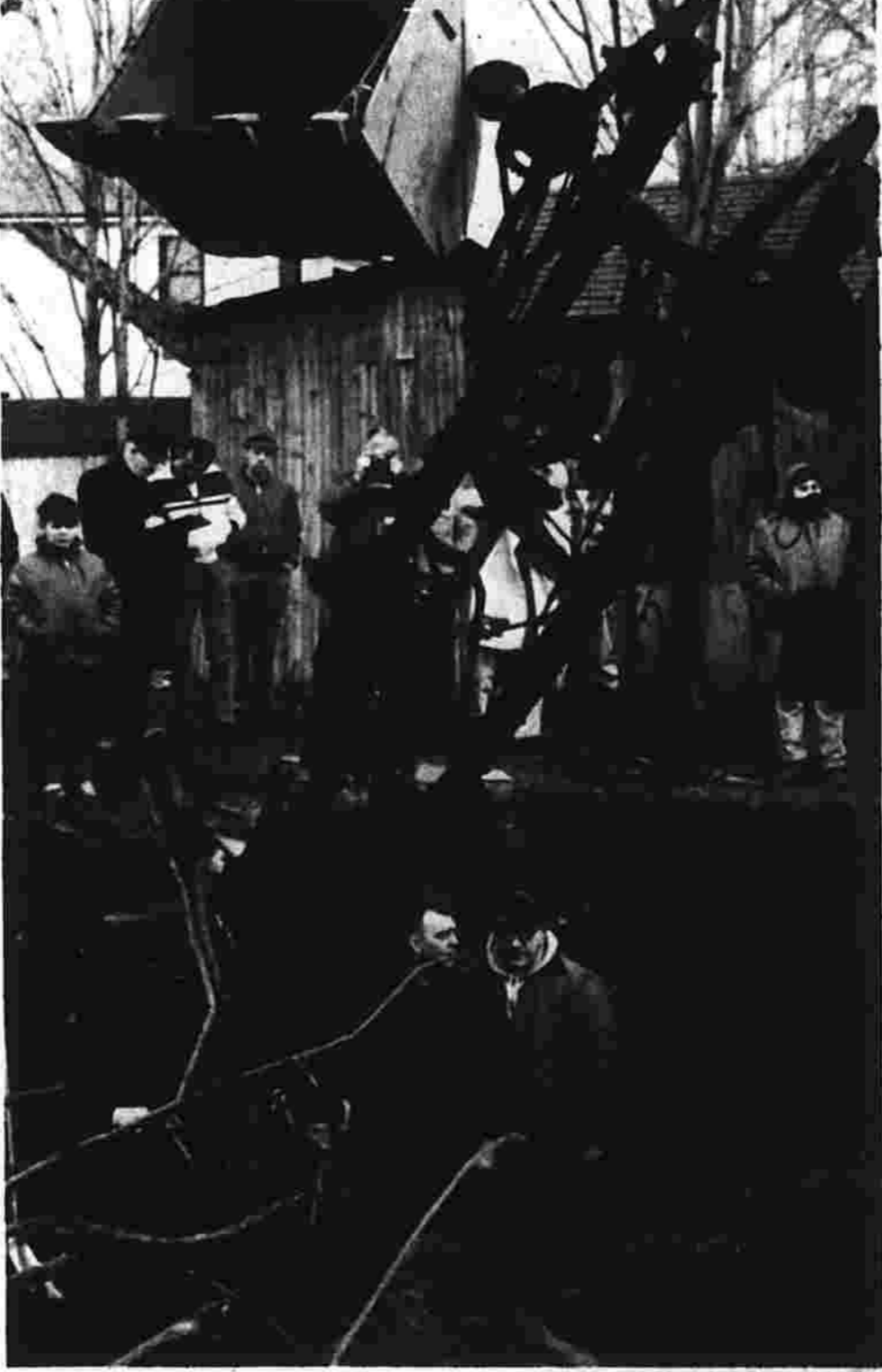
Watching Herbert O'Dette of Storrs, at the controls of the backhoe, lift the 1912 Metz chassis from the site of a former blacksmith shop at Adams St. and Tolland Tpke. are antique buffs William Bedford of Willington, partially hidden; William Stewart, in charge of restoration at the Antique Auto Museum on Slater St.; and Walter MacGregor of East Windsor, a charter member of the Hinckley Carriage Club. Another worker, Walter Sodyan, 52 Gerard St., was elsewhere when the picture was taken. Visible at the top are the chain drive and shaft, which propelled the car. (Herald photo by Pinto)
